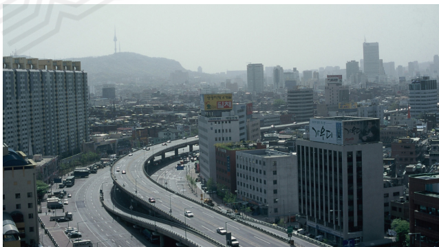
[Figure 6] Before demolishing the elevated expressway above the Cheonggyecheon in 2000
