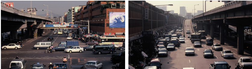
[Figure 5] Elevated Expressway above the Cheonggyecheon in 1995
