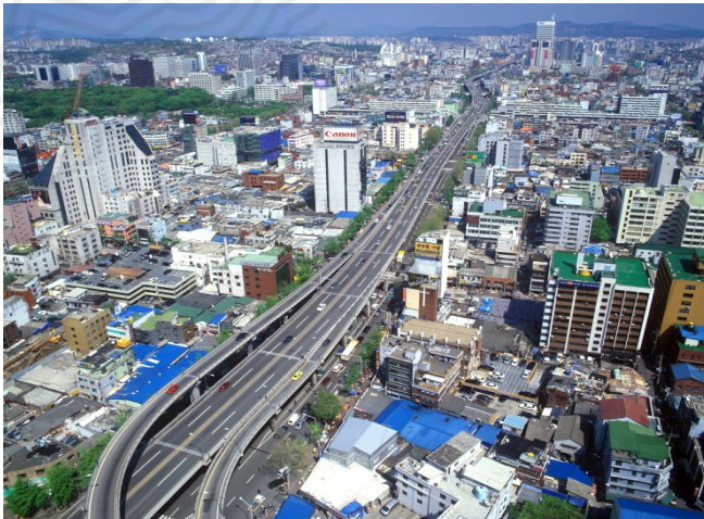
[Figure 7] Before demolishing the elevated expressway above the Cheonggyecheon in 1990s
