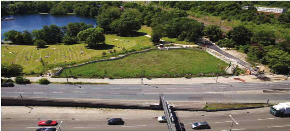
Retention ground filter at Halensee purifies the heavily soiled rainwater from the motorway
